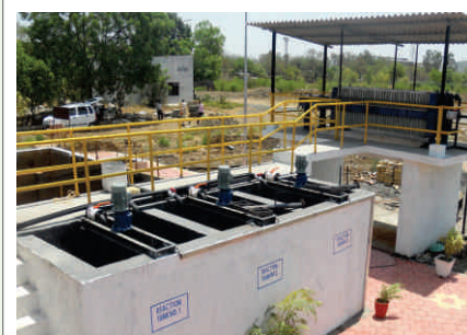
M/s Tata Steel Ltd. (Wire Division) Pithampur
